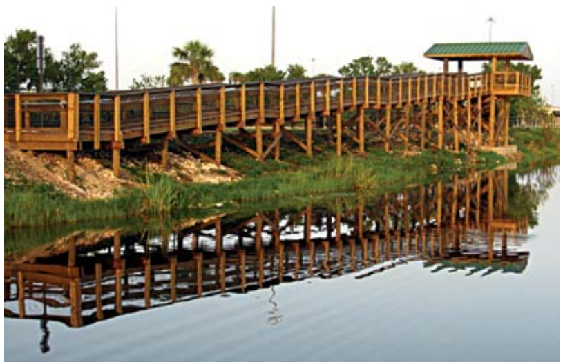
Top to bottom: Babcock Webb WMA's ADA-accessible shooting range section; a wheelchair or walker can easily be maneuvered inside a blind at Andrews WMA; Everglades WMA provides a newly constructed overlook at a rest stop along I-75.
